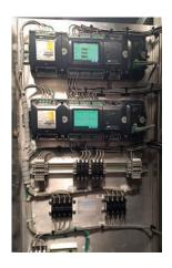
The BFM-II is ideally designed to upgrade existing substations with electro-mechanical relays to provide real-time information and management lacking in these highly reliable devices.
